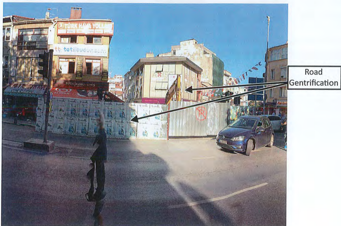
Figure 24: Road Improvement Construction in Site 9 (self-taken photograph)
